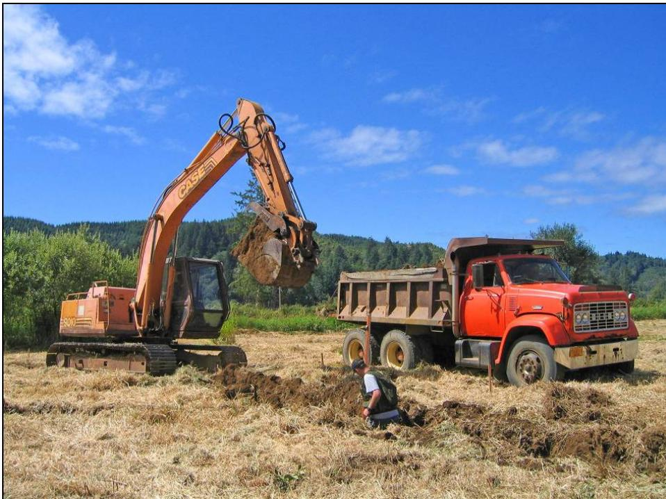
Photo A3. August 14, 2007: Excavation of pilot channel at site S65. Jeffrey Jones measures channel depth while Nathan Large operates the excavator. Photo by Laura Brophy.
