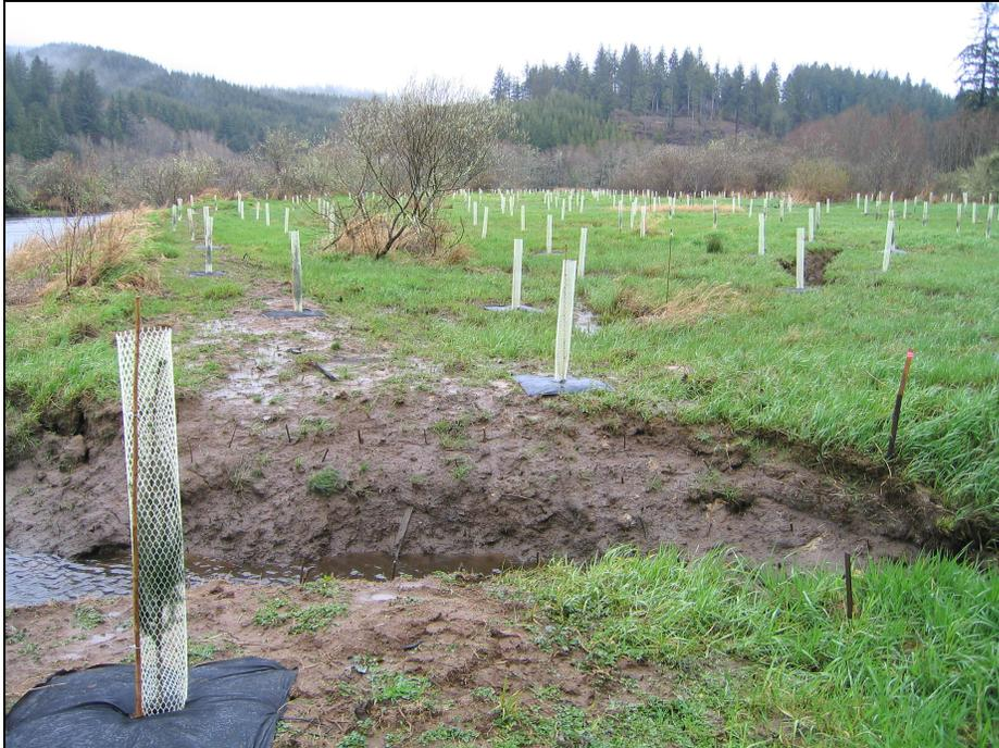
Photo A6. March 17, 2008: Site S65 north-facing view of dike breach and former pasture; partial dike removal and extensive shrub and tree plantings can be seen (white Vexar tubes). Photo by Laura Brophy.
